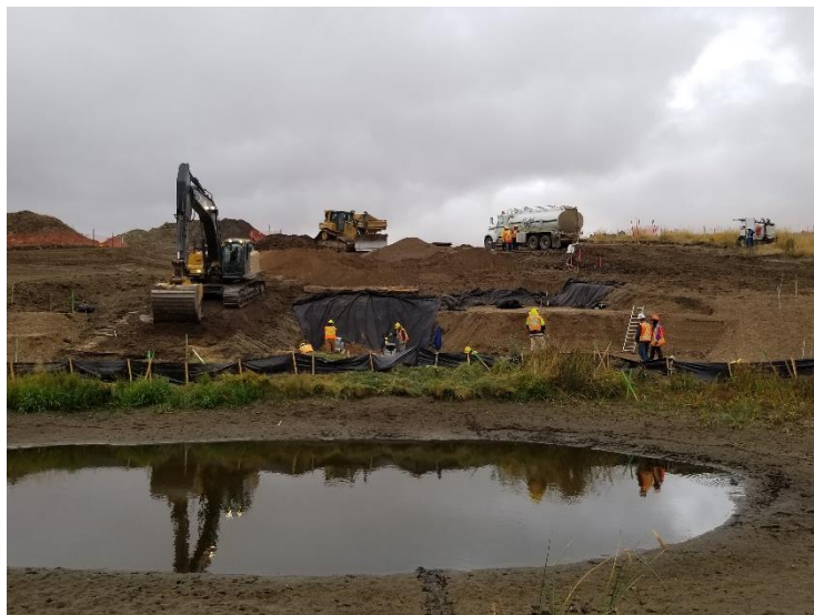
Topsoil completely over and dozer levelling.
