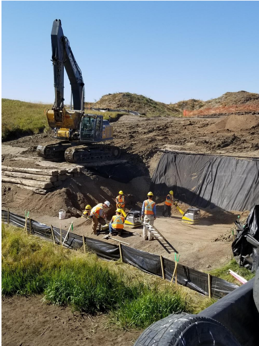
At High Hill creek they construct diversion berms (Panels) to correct slope and future sloping.
